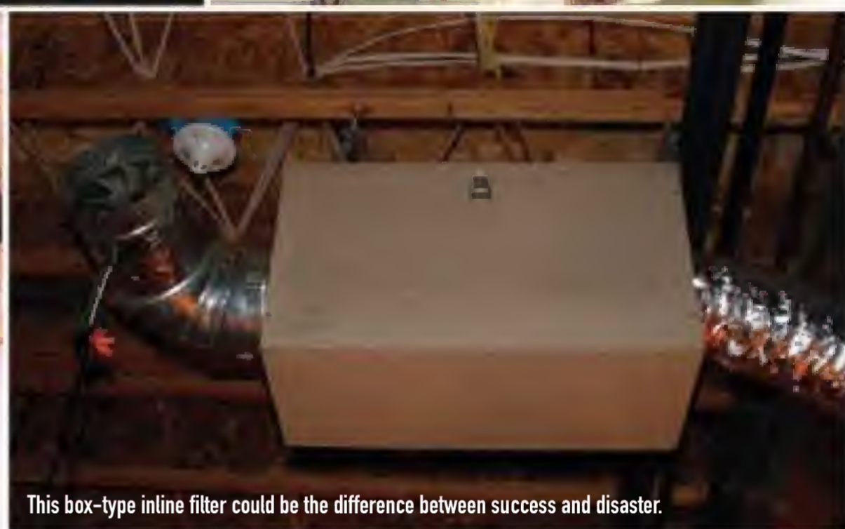
Always attach tubing securely using flanges to avoid air and odor leaks.
